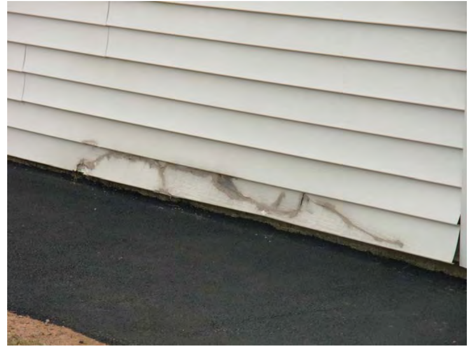
6. Vinyl siding - spot damage
