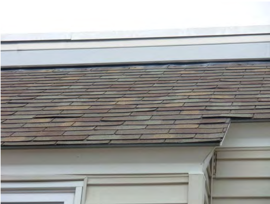
7. Spot lifting of mansard roofing shingles
