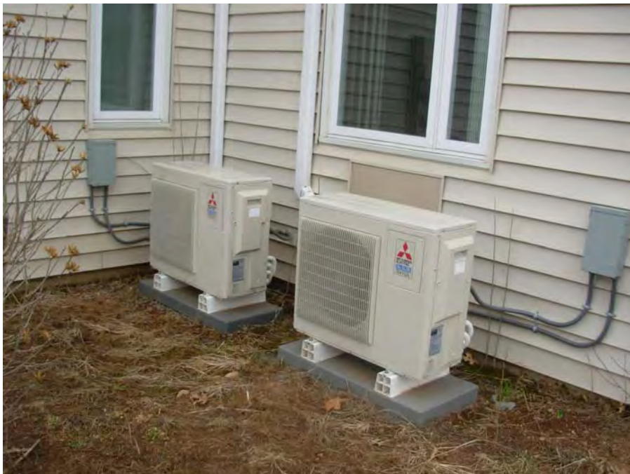
15. Heat pump HVAC system exterior condensers
